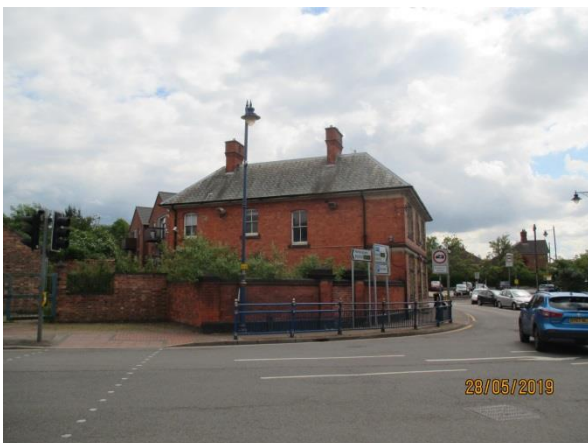
North elevation of the police station building
